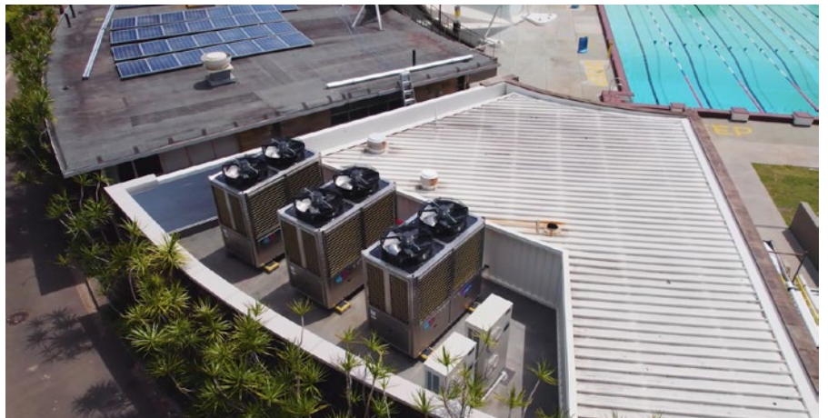
Electric heat pumps replacing gas at Victoria Park Pool. Credit: Supplied by Image Air Conditioning
