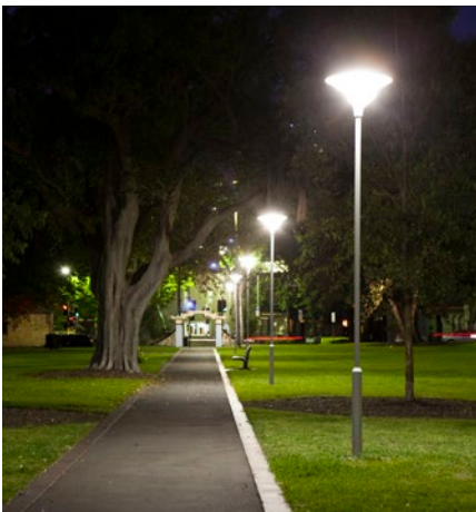
LED lighting in Alexandria Park Credit: Jamie Williams
