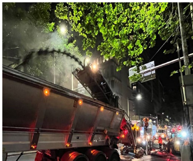
Replacing the road surface on Clarence Street with asphalt containing recycled materials to lower its embodied carbon. Credit: Matt Formica
